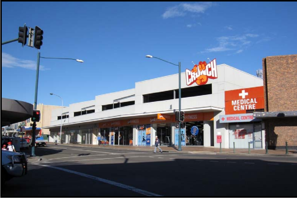
Figure 2: Photograph of existing development frontage to Scott Street
