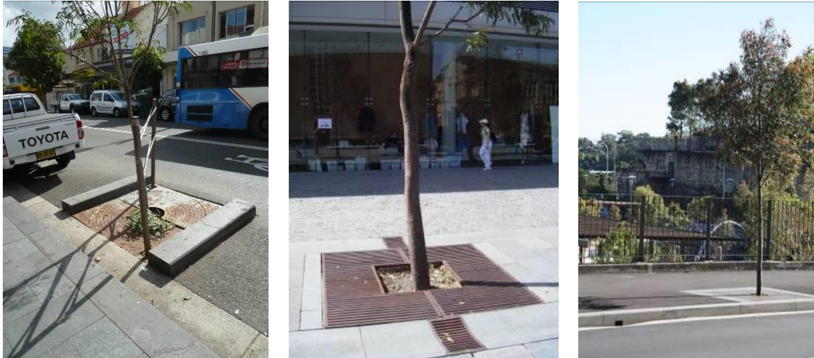
Figure 11: WSUD in Street Tree pits – Redfern St (left), Sydney University (centre) and Pirrama Park (right) (Photos: Alluvium).
