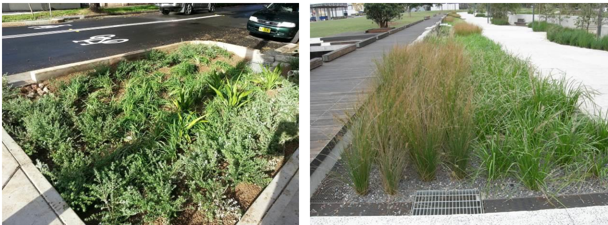
Figure 12: WSUD rain-gardens in Sydney – Telopea St, Redfern (left) and Pirrama Park, Pyrmont (right), (Photos: Alluvium).
