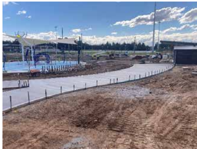
Stante Reserve – works underway
