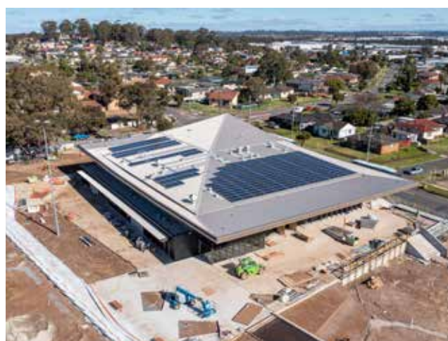
Phillips Park - works underway
