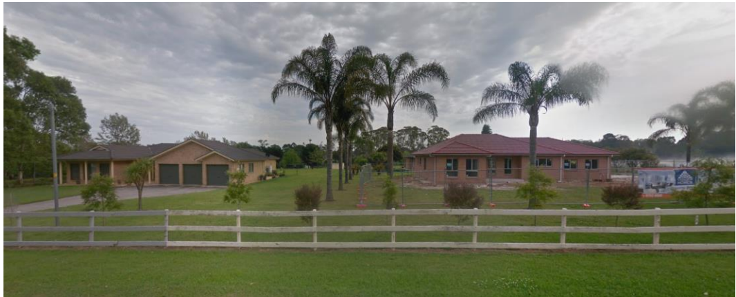
FIGURE 71: DUAL OCCUPANCY CONSTRUCTION IN ROSSMORE
