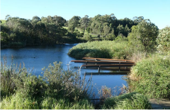
Figure 92: Sydney Park incorporates a water harvesting function, collecting storm water from the surrounding streets, allowing it to move through the parkland and slowly be purified of pollutants through a process of biofiltration. (Source: Arterra)
