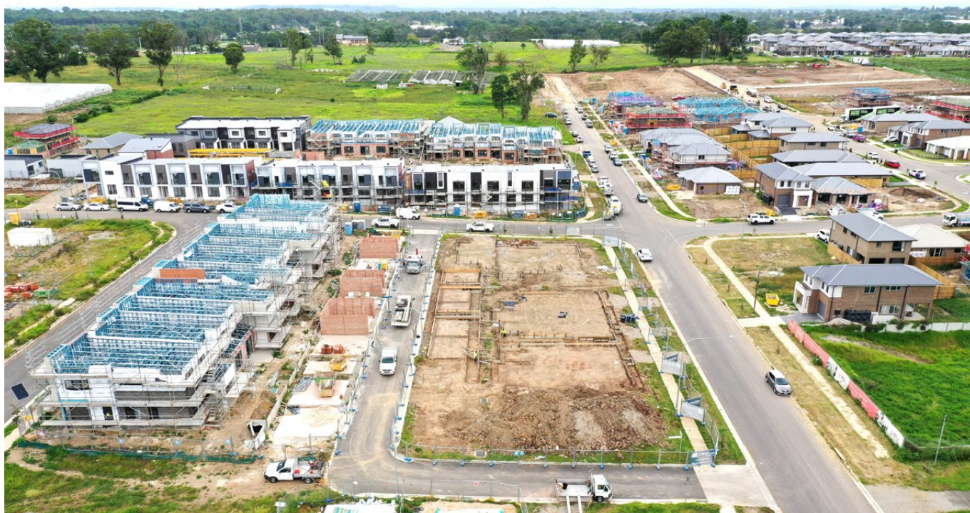
Figure 30: Current patterns of urban release lands, are often not conducive to the protection of existing trees or the establishment or expansion of tree canopy. Small sized allotments, in combination with the tendency to build very large residences, results in extremely limited opportunities for tree planting on private property. (Source: Liverpool City Council)
