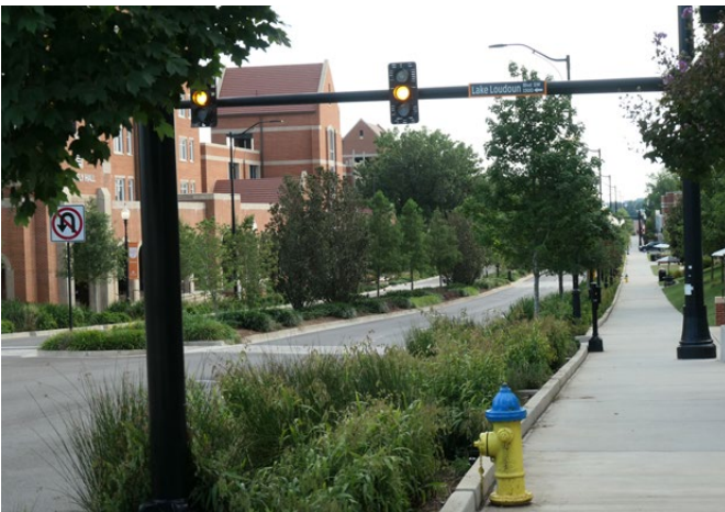
Figure 93: Extensive rain gardens and passive irrigation for street and tree planting in Knoxville, Tennessee. (Source: Arterra)
