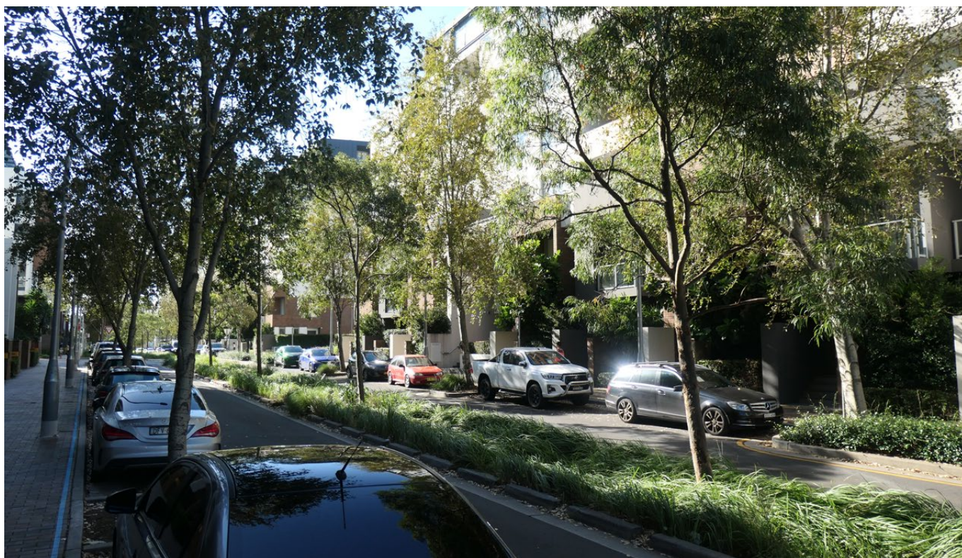
Figure 96: Harold Park, Sydney where median swales and rain gardens serve to treat stormwater and passively irrigate extensive tree planting. (Source: Arterra)
