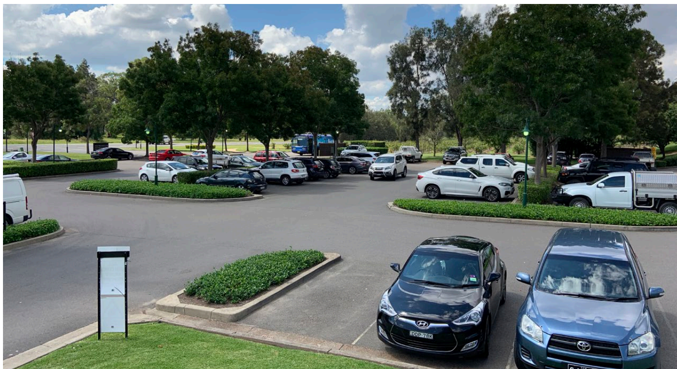
Figure 108: Incorporation of trees in car parks, provides very welcome shade for cars as well as reducing heat loads and re-radiated heat from pavements. Lack of tree planting and shade to car park and inappropriate space and physical provision for trees should no longer be accepted. (Source: Arterra)
