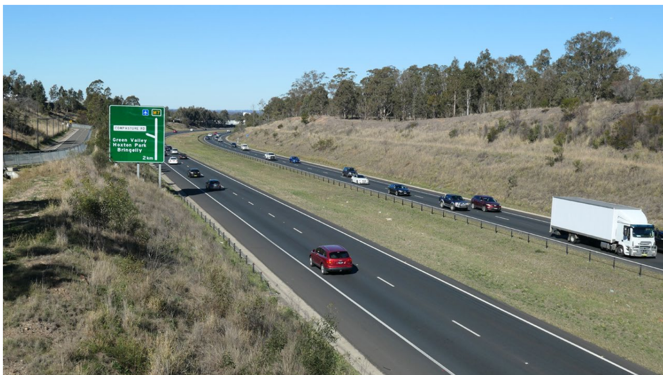
Figure 22: Many of our major motorways are controlled and managed by the state government rather than Council. Due to the nature of these corridors, many of the more recently constructed motorways actively contribute to our canopy cover and habitat connectivity through extensive roadside tree planting. (Source: Arterra)
