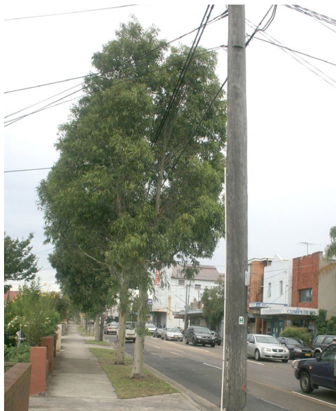
Figure 62: Trees and overhead power lines can co-exist if managed well and overhead cables are converted to ABC before planting reaches mature heights. A particularly successful outcome is demonstrated along Gardners Road in Rosebery. (Source: Arterra)
