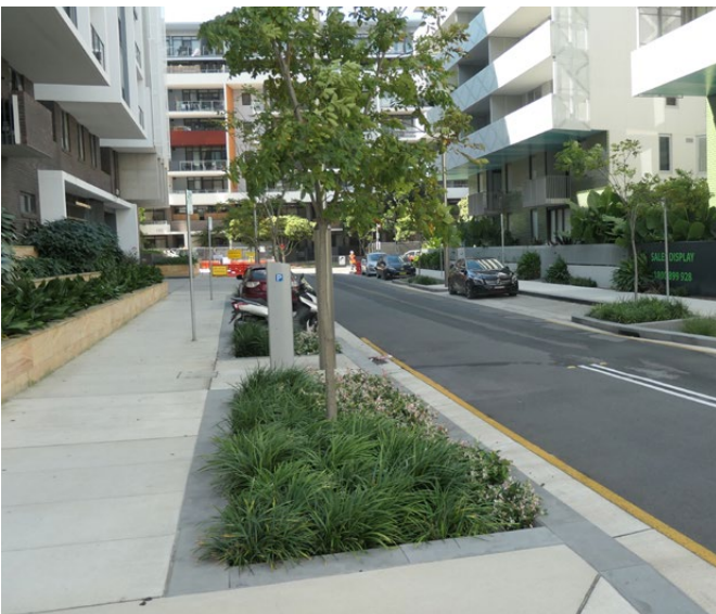
Figure 94: Permeable and street side rain gardens can be used extensively in public spaces to allow water to be retained in the landscape, replenish the water table and provide a passive, economical and sustainable source of moisture for tree growth. (Source: Arterra)
