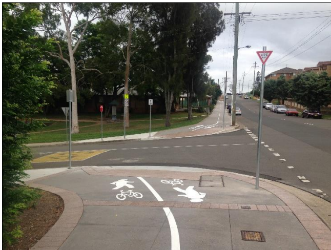
Figure 2-6: Off-road shared pathway with markers and signposting, Mill Road, Liverpool
