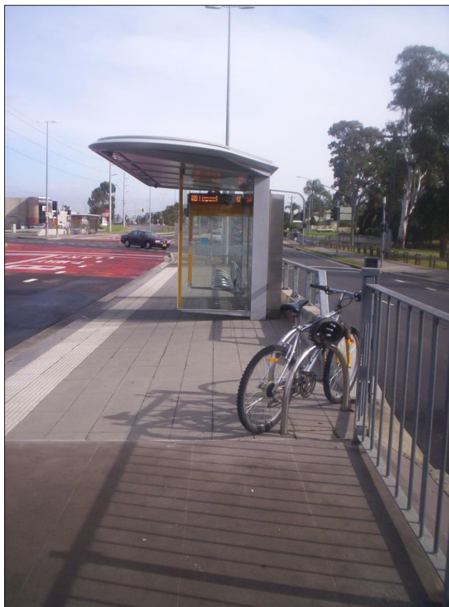
Figure 2-9: Parking facilities on the Transitway, Maxwells Transitway Station.
