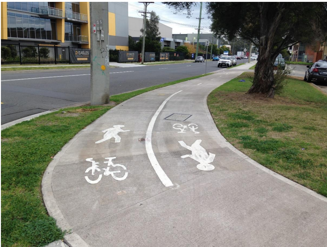
Figure 2-8: Off-road shared pathway with markers and signposting, Jedda Road, Prestons
