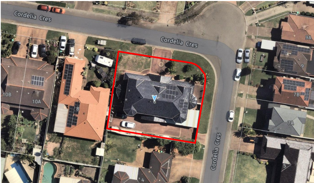
Figure 1: Aerial view of the site (Source: Nearmap)
