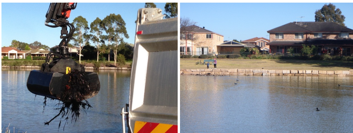
Photos showing sediment removal and bank protection works undertaken.
