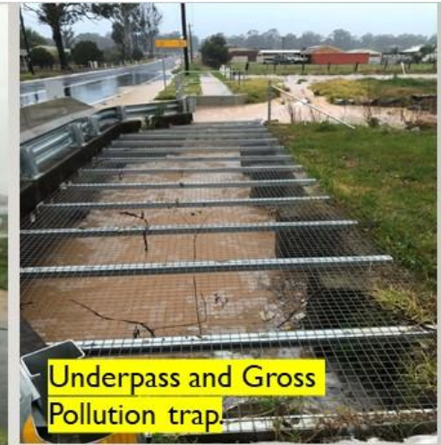
Underpass drains blocked causing road flooding.
