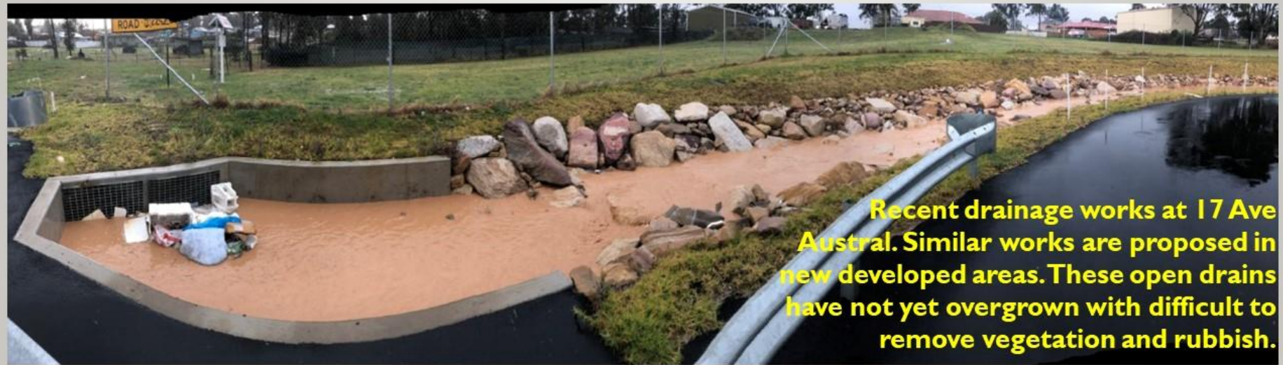
Underpass and Gross Pollution trap
