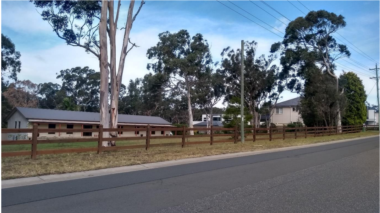
Figure 7 Looking south-east toward Lot 5 Pleasure Point Road
