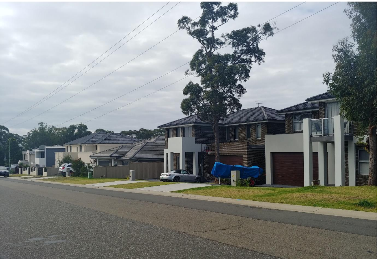
Figure 6 Looking north-east at the no.72 dual occupancy development and further down Pleasure Point Road
