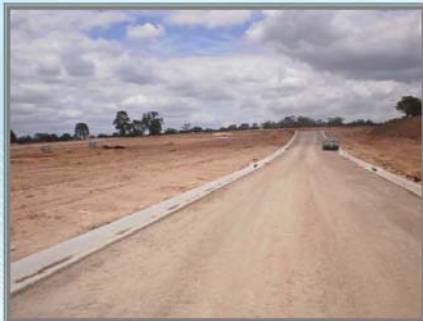
Subdivision works at Elizabeth Hills
