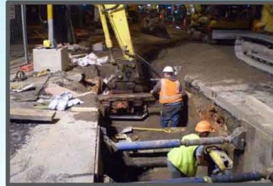
'George Street trunk drainage – drainage construction works at night'
