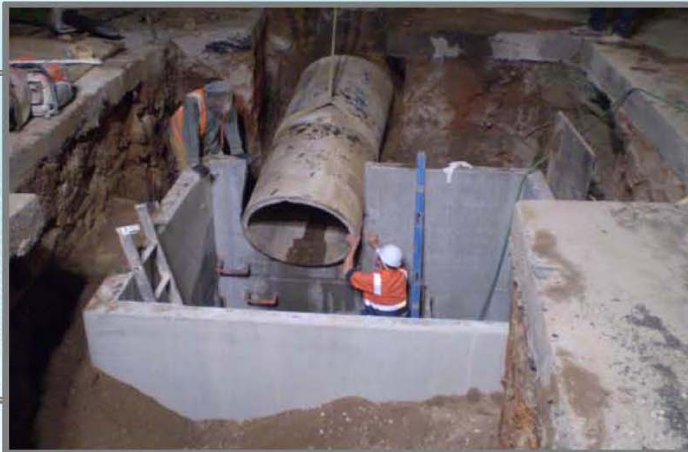
City Centre Trunk Drainage
