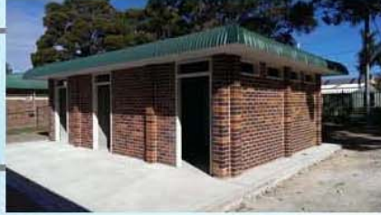
New amenities building at Rosedale oval
