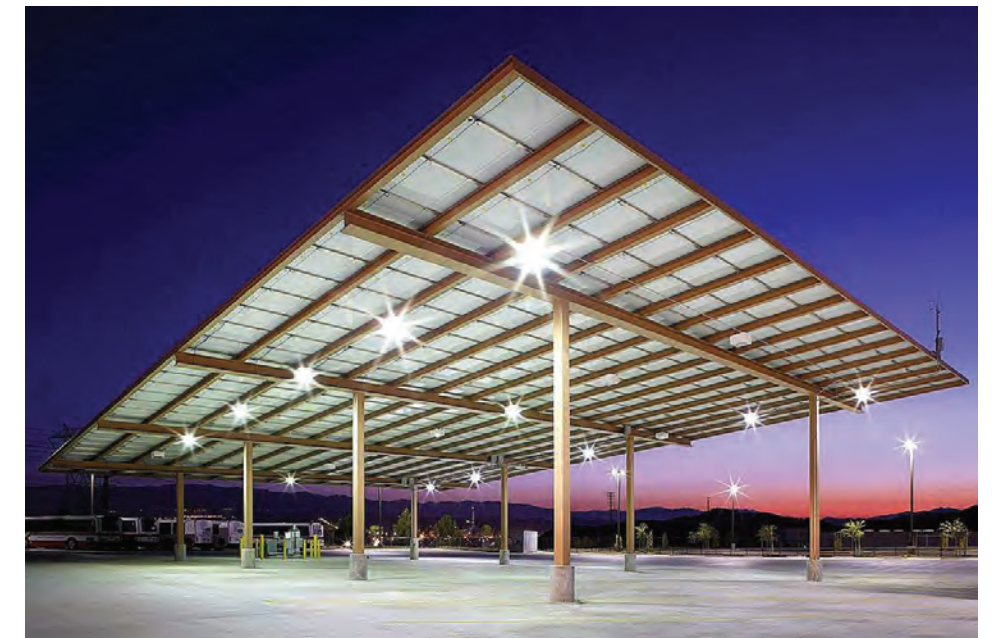
SOLAR PANELS TO LEVEL 4 CARPARK ROOFS
