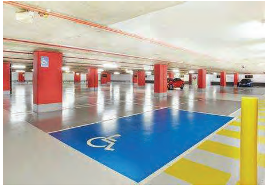
ACCESSIBLE SPACES CLEARLY IDENTIFIED AND IN ACCORDANCE WITH AS1428.1
