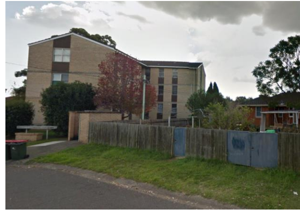
Public housing apartments in the eastern part of the 216 District
