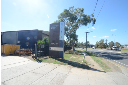
View of the site frontage at Newbridge Road.
