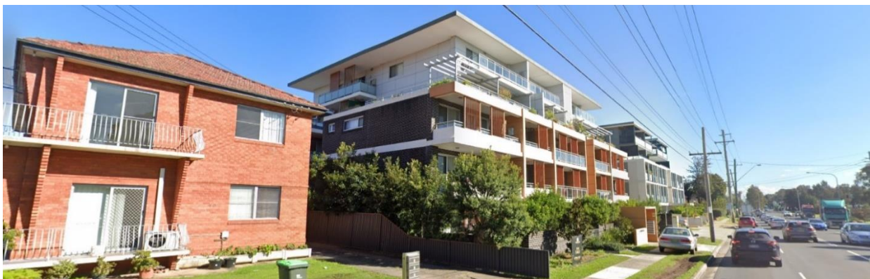
Figure 12: View of a two separate 5 storey residential flat buildings where levels 4 and 5 are further setback from the streetscape than levels 1 -3, reducing the bulk and scale of the development. Each development is across 2 allotments (Approximately 30m width).
