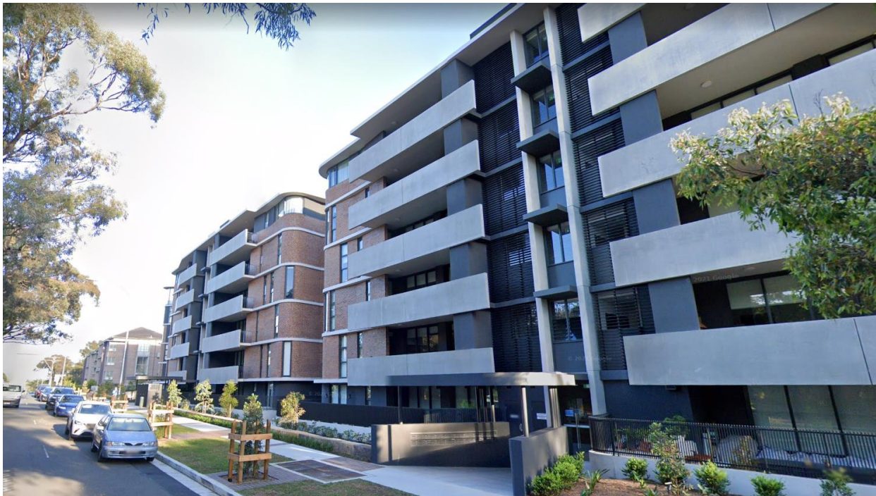
Figure 13: View of a two separate 6 storey residential flat buildings built closer to the street setback and with no indentation to upper levels increasing the bulk and scale. Each development is approximately 45m width.
