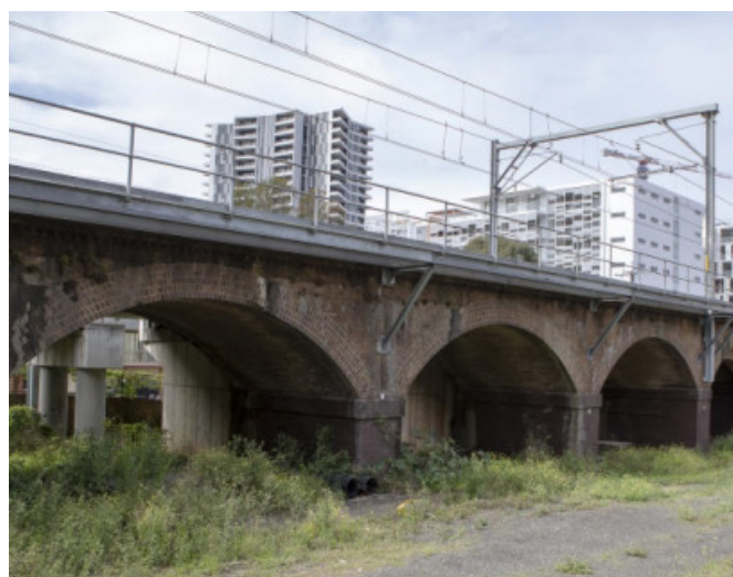
Figure 6.273 Liverpool Railway Viaduct (Liverpool City Council)
