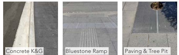
Figure 6.287 Images of Core Paving (Bluestone), Kerb & Gutter and Ramps
