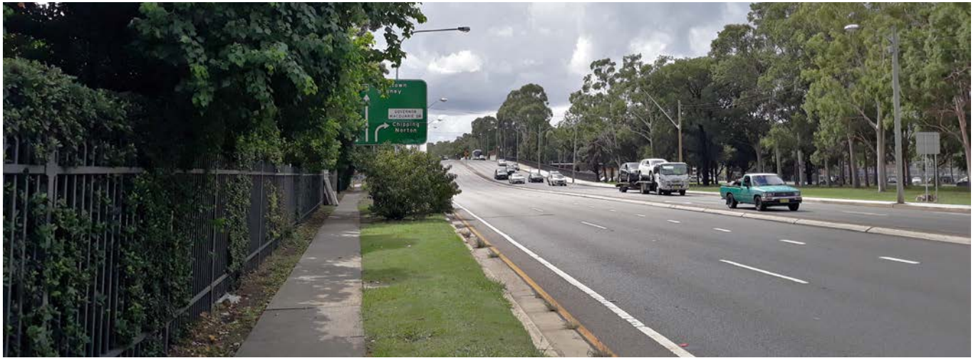
Figure 8.341 Hume Highway eastern side, close to Sheahan Pathway, looking east.
