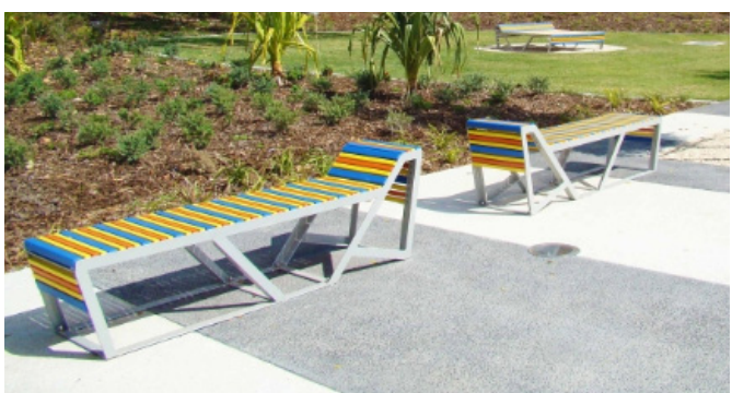
Figure 6.302 Recycled plastic street furniture designed by AECO, M for Southport Broadwater Parklands, Gold Coast.
