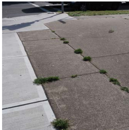
Figure 8.331 Pavement detail. Bigge Street north section close to Campbell Street.
