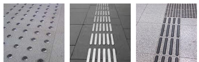
Figure 6.291 Images of Tactile Indicators on Paving
