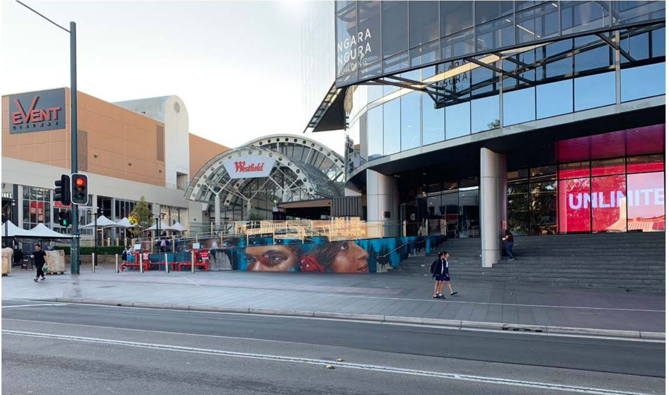
Figure 6.231 Western Sydney University Forecourt - Before (Liverpool City Council)
