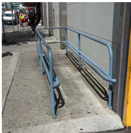
Figure 8.355 Detail of trolley bay on George Street's south side, close to Elizabeth Street.
