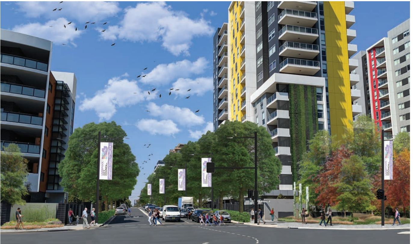
Figure 6.207 Bigge Street (North) Gateway - After (Liverpool City Council)
