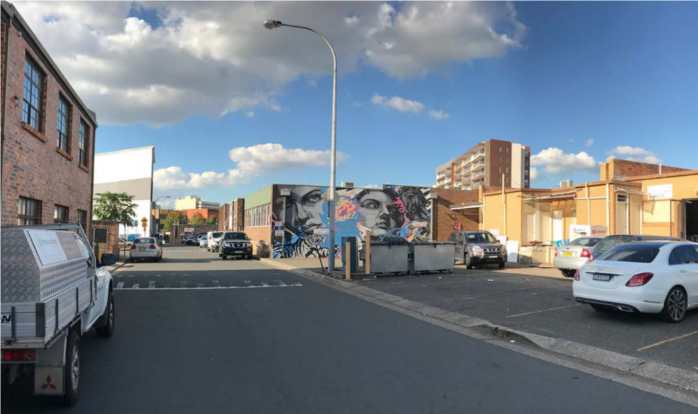
Figure 6.203 Norfolk Serviceway Upgrade - Before (Liverpool City Council)
