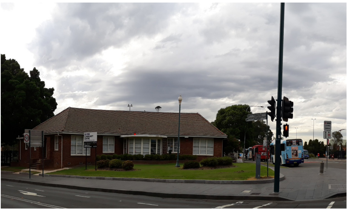
Figure 6.260 Dr. Pirie Community Centre, Forecourt - Before (Liverpool City Council)
