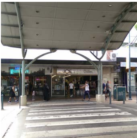
Figure 8.394 Pedestrian crossing Macquarie Street with rooftop cover.
