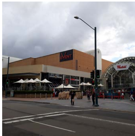
Figure 8.384 Aspect of Macquarie Mall from the intersection with Elizabeth Drive.
