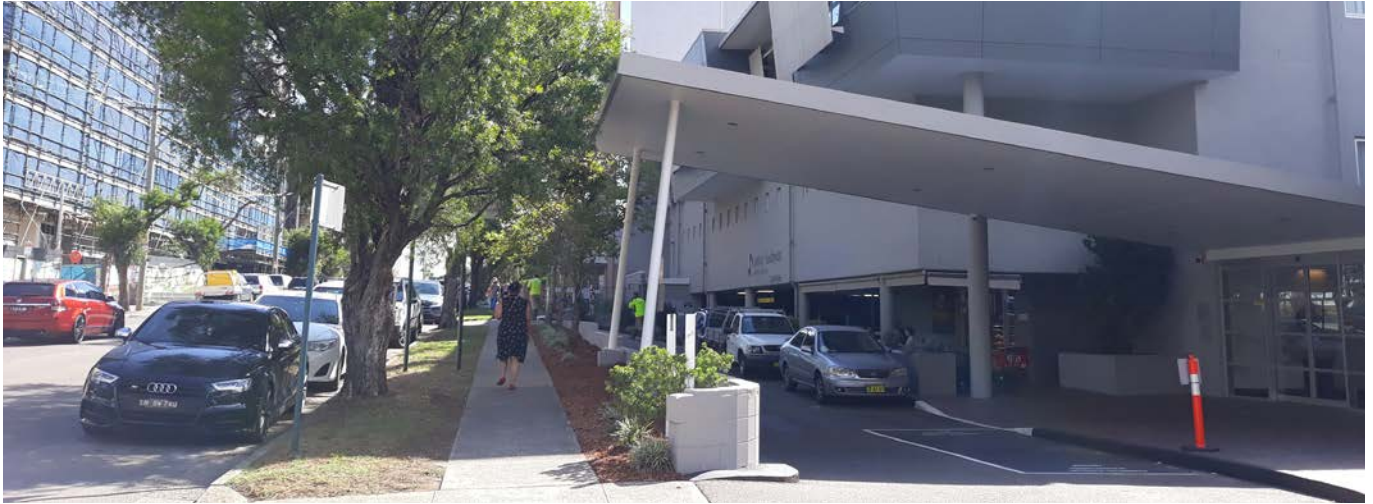
Figure 8.329 Sydney Southwest Private Hospital Entrance near Tindall Avenue.
