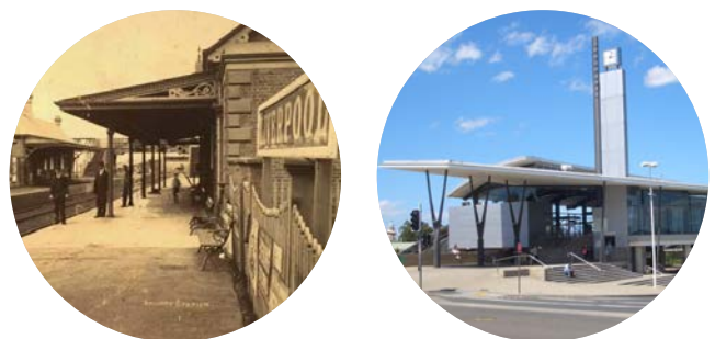
Figure 6.256 Liverpool Station Past & Present (Liverpool City Council)
