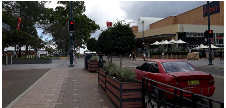
Figure 8.386 Detail of planting box on Elizabeth Street's south side, view from the entrance of Macquarie Mall.
