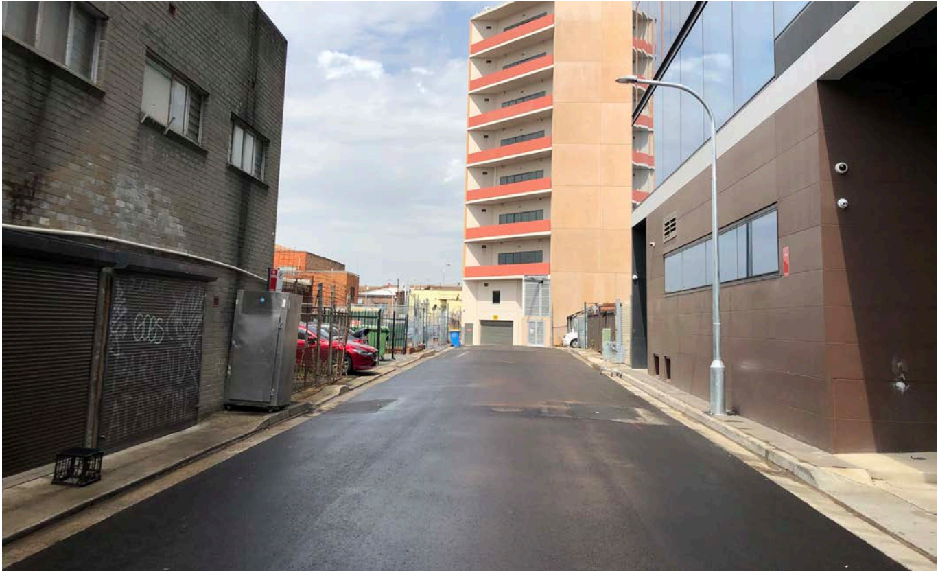
Figure 6.317 Railway Serviceway - Before (Liverpool City Council)
