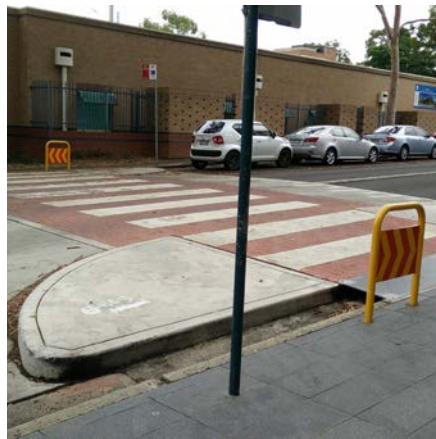
Figure 8.361 Pedestrian crossing Campbell Street east side, close to Forbes street.
