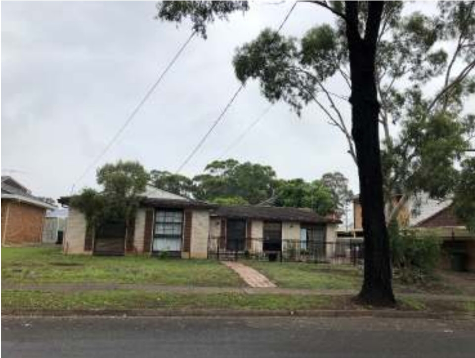
Figure 3: View of existing dwelling from Kalimna Street
