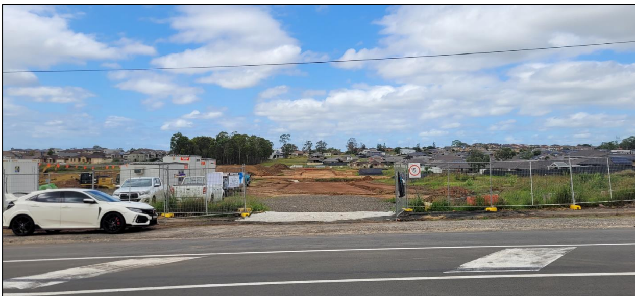
Figure 5 – View of the site from Southern Cross Avenue
