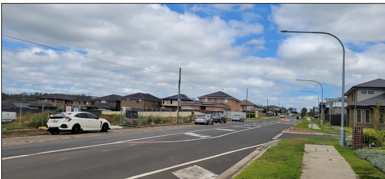
Figure 6 – View of the intersection of Southern Cross Avenue and Briggs Avenue, the location of the future roundabout
