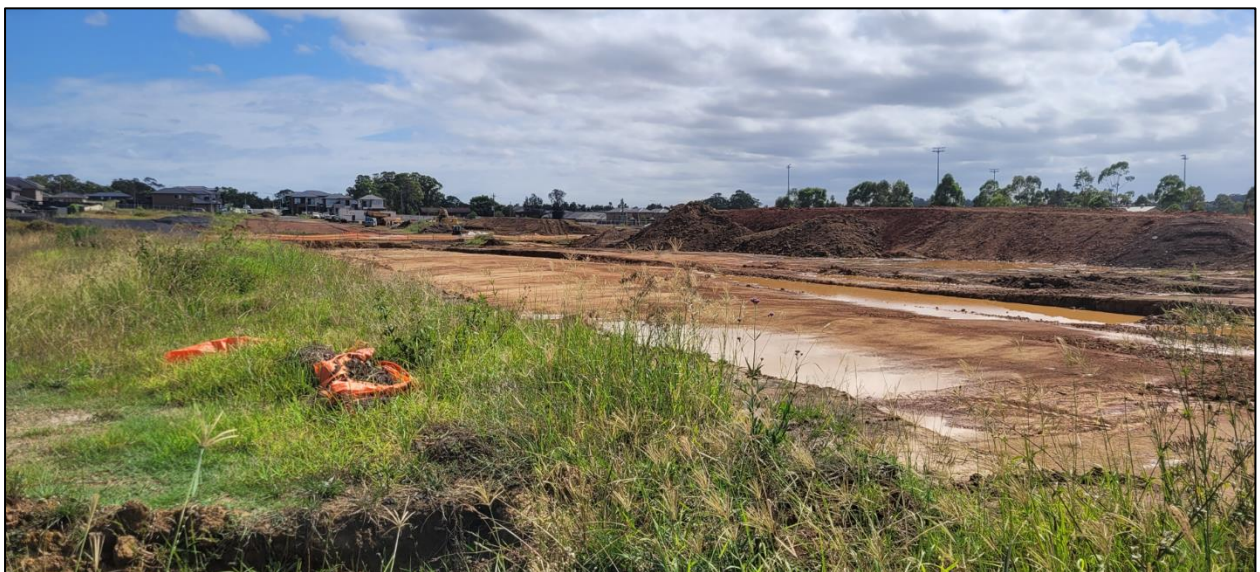
Figure 4 – View of drainage work from
