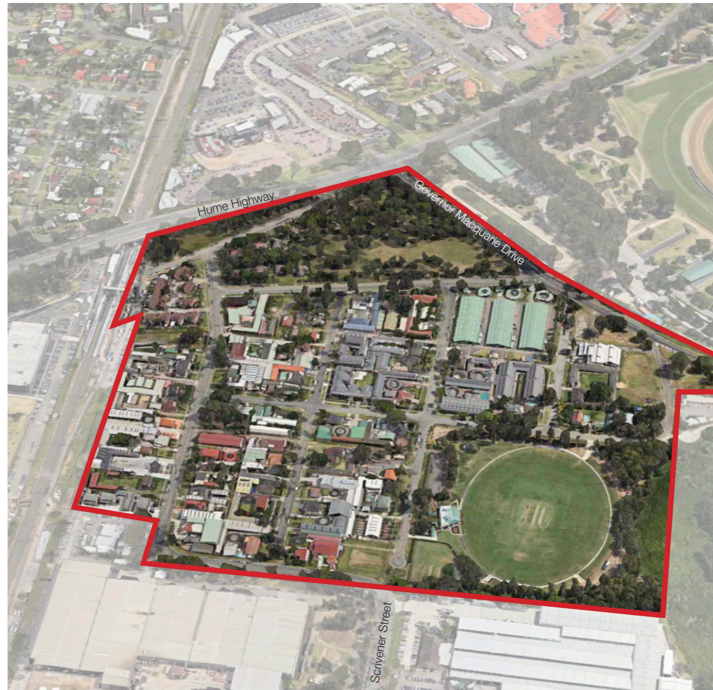
Figure 1: Aerial view of the Warwick Farm Precinct
