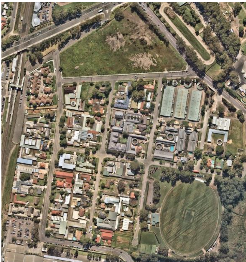
Figure 1: Aerial view of the Warwick Farm precinct NB: 240 Governor Macquarie Drive, depicted at the top of the picture, is not included among the lots subject to the planning proposal. Source: Nearmap 15 April 2020
