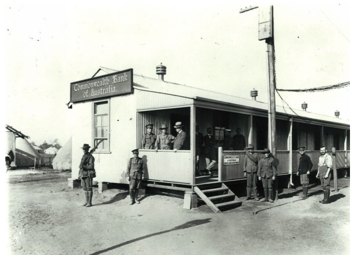
Commonwealth Bank at Holsworthy Army Barracks, 1914—1918, Item from Fonds: Heritage Library Photograph, HL002901-1, Liverpool City Council.
