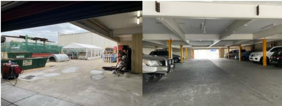
Figure 10: Site Inspection photos of the basement parking and rear of the site
