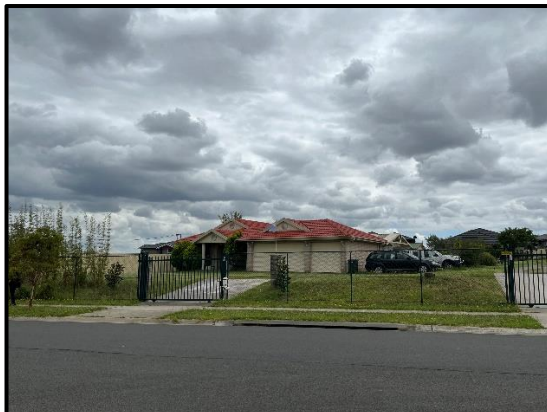
Figure 3: The existing dwelling located on the western portion of the subject site.
