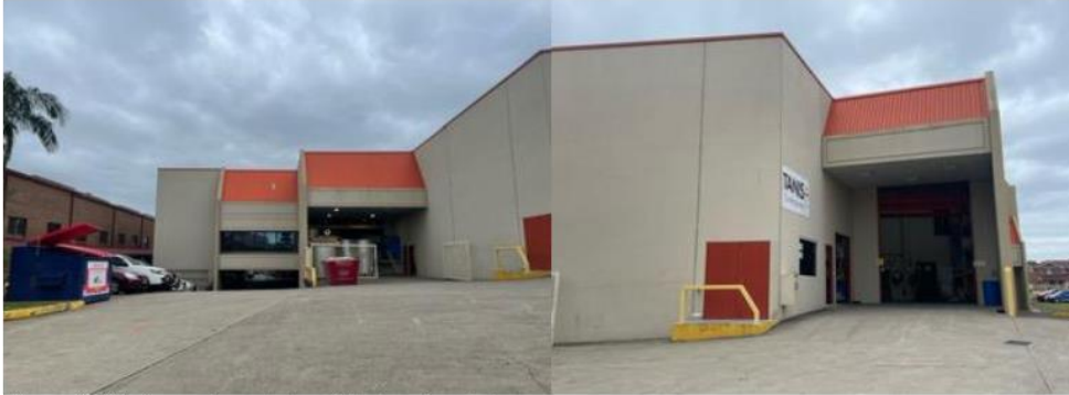
Figure 9: Site Inspection photos of the loading docks
