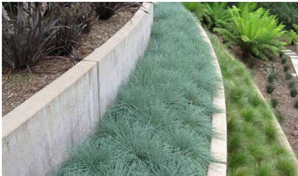
Terracing is enhanced by planting.
