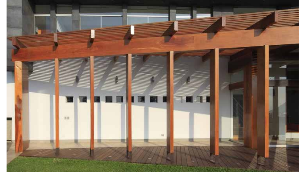
Shade structure adjoining building.
