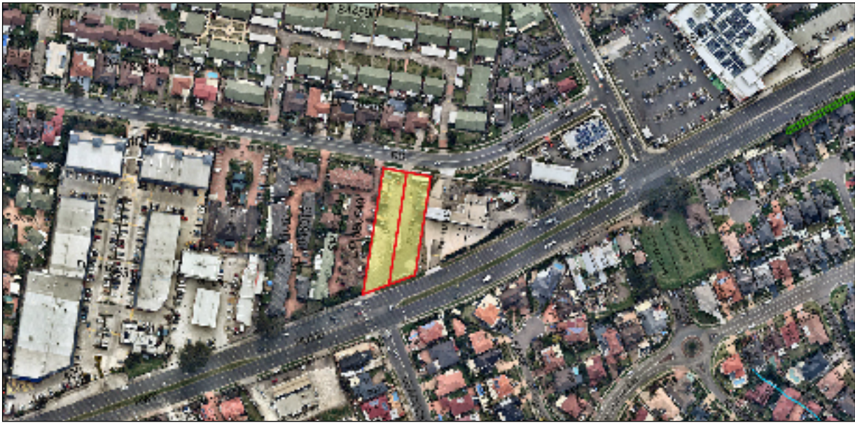
Figure 1: Locality Surrounding 619-621 Hume Highway, Casula (Source: Geocortex)
