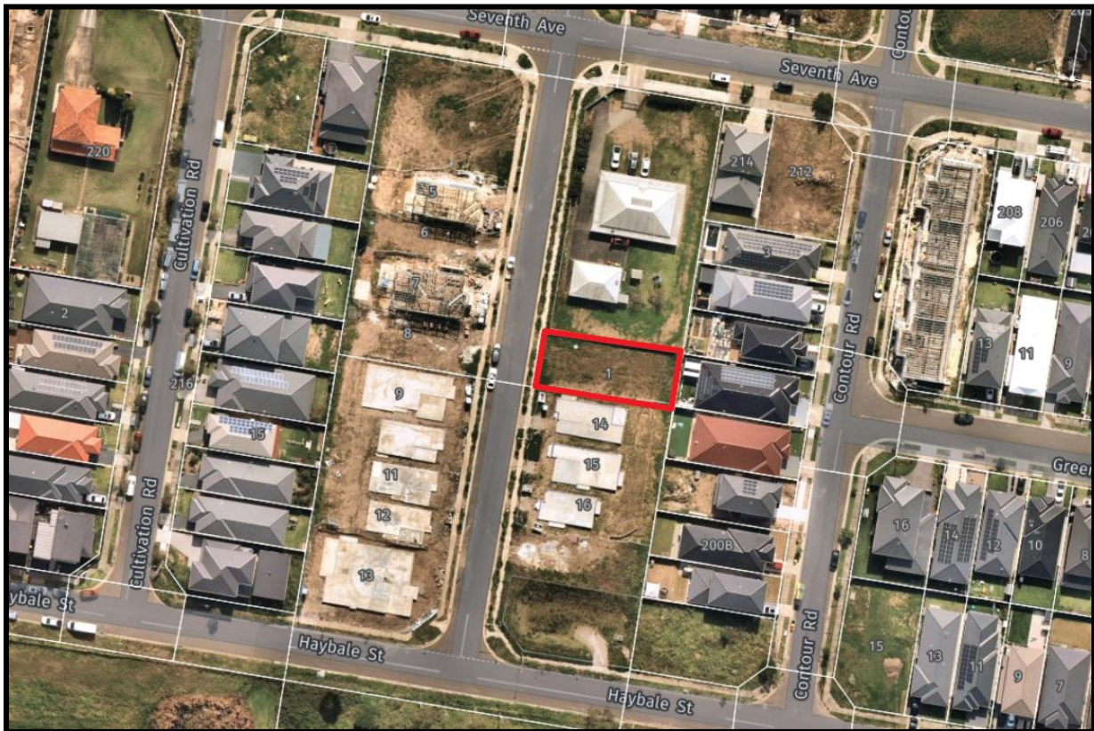
Figure 3: Indicative aerial view of the site (Source: Nearmap)
