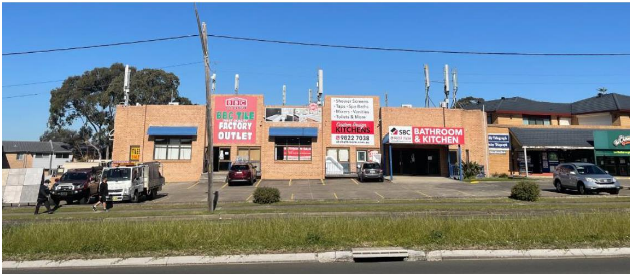
Figure 2: The existing Telstra communications facility located on the roof of 560 Hume Hwy, viewed from the Hume Highway.
