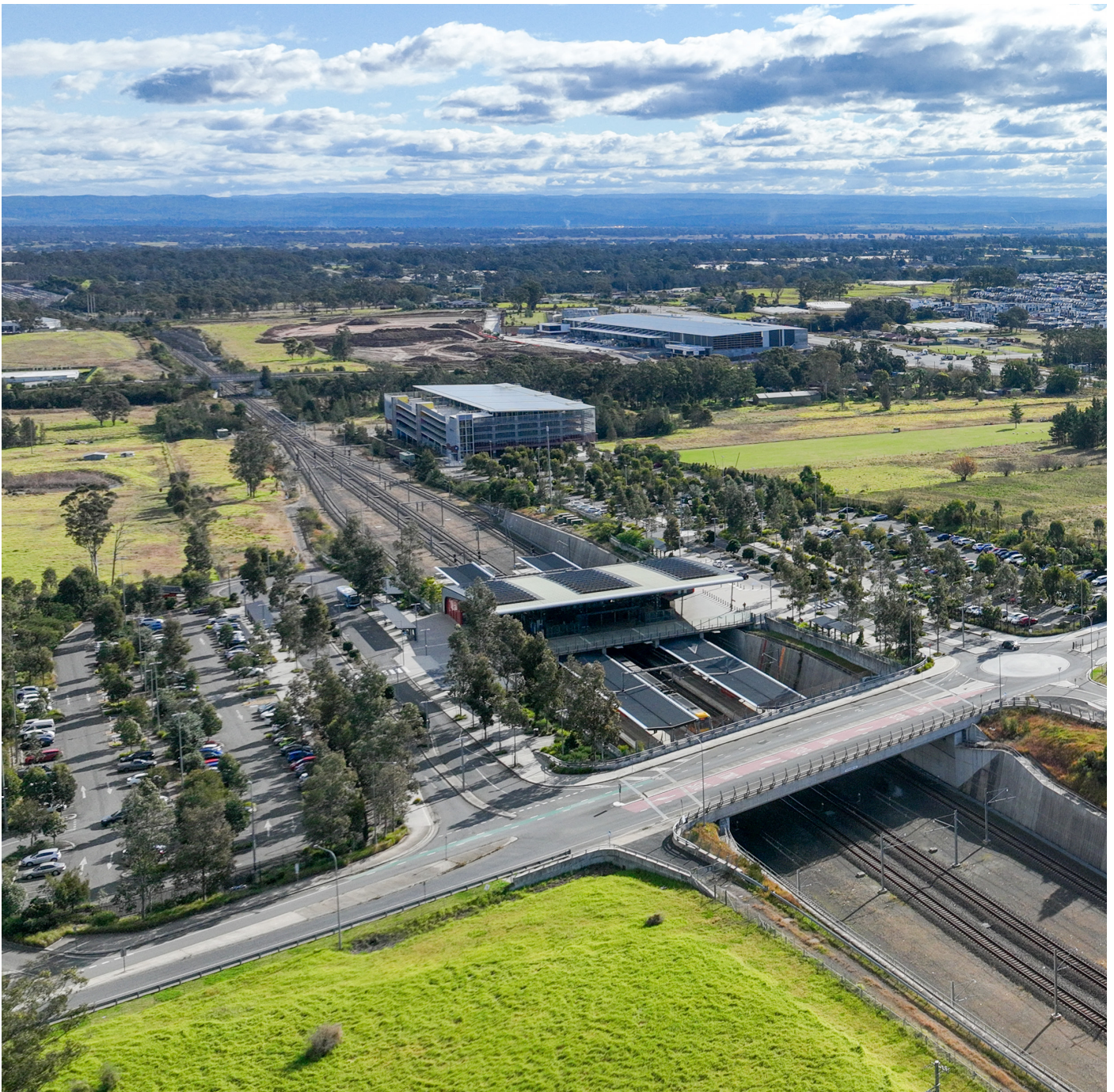
Figure 2: Rickard Road, Leppington Train Station and the commuter car park
