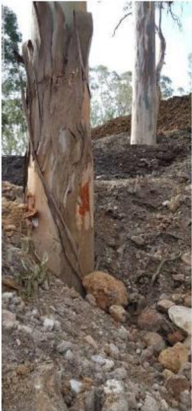
Image 7 - Soil material had been placed directly around the trees displaying preservation numbers to a depth of several metres high
