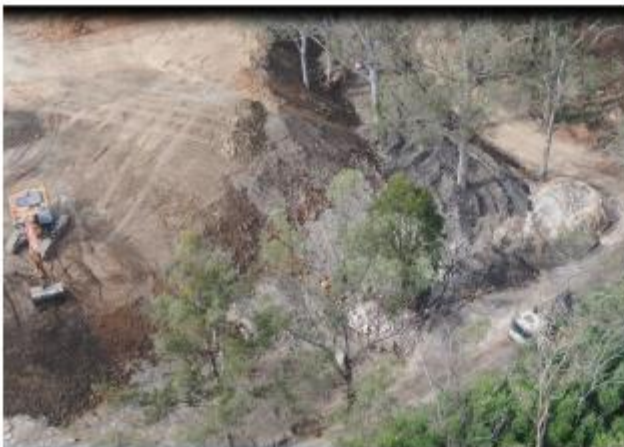
Image 5 - Aerial view of excavator operating on Western batter
