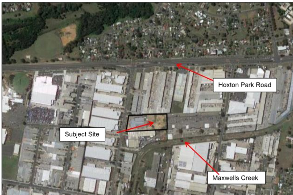
Figure 1: Aerial view of Subject site and immediate surrounding locality
