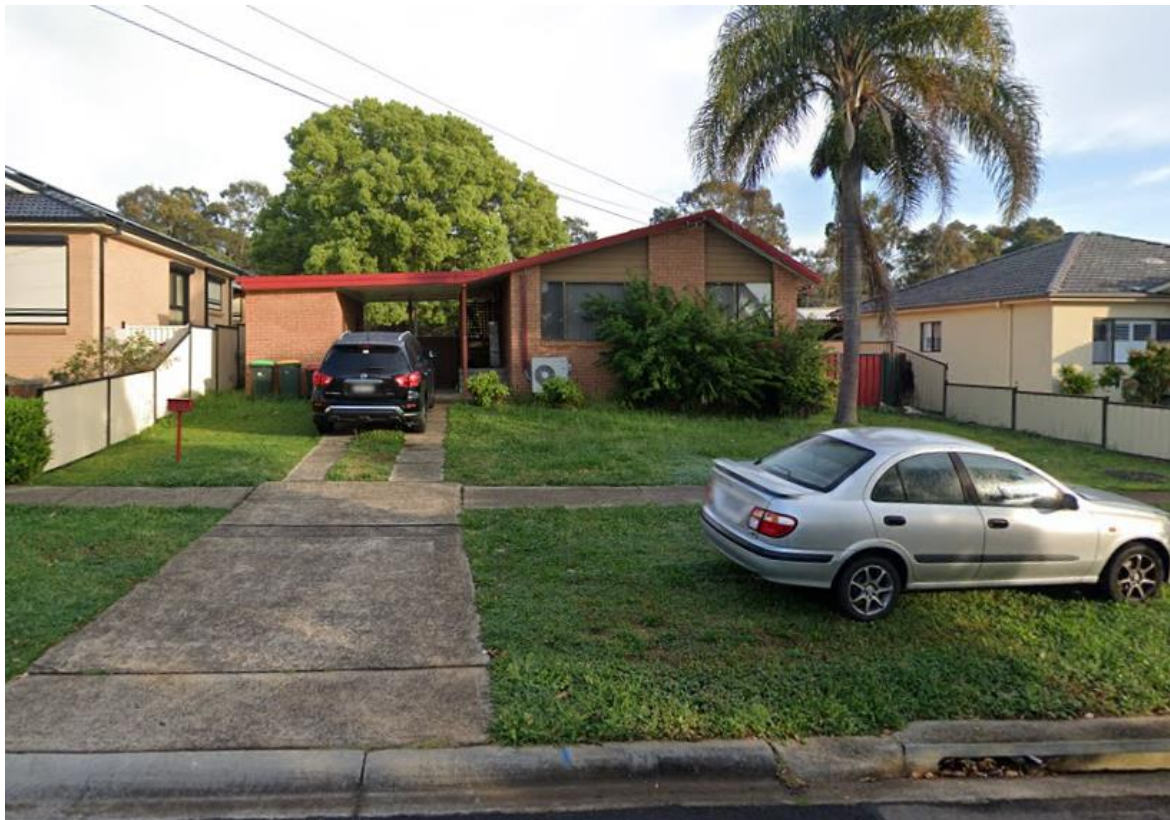
Figure 2: View of the site as seen from Artillery Crescent consisting of a single storey brick detached dwelling with a brick garage and a carport attached to the side (Source: Google Street View).
