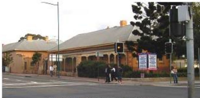
Former Liverpool Courthouse (State significant)
